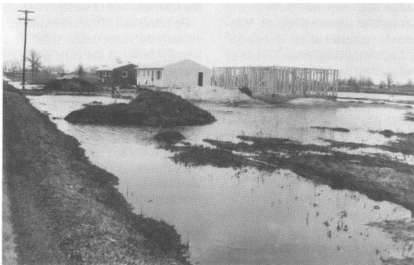
FIGURE 6.5 Dewatering, surface and subsurface drainage, is required to make this land suitable for both building construction and cropping. (Photograph courtesy Soil Conservation Service, USDA.)
