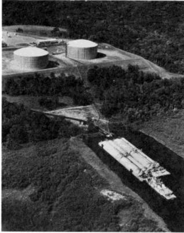
Figure 3. Ammonia Storage Terminal at Pine Bend, Minnesota.
